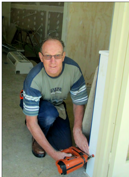
Stephen working on the classroom
