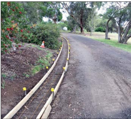
Form work before drains and hot mix
