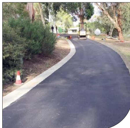
Completed road and dish drain
